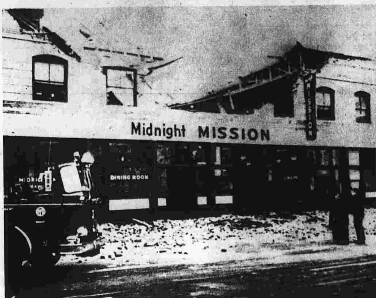
Rubble from a partially collapsed building at the Midnight Mission in downtown Los Angeles marks the area where two men were killed this morning when an earthquake rocked the area. (AP Photo)
